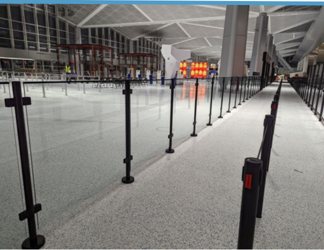
Designed from scratch, the post and glass partitions ultimately provided the architect's vision on the owner's budget. A win-win.
