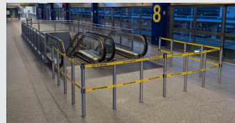
Retractable belt barriers can be implemented during maintenance.
