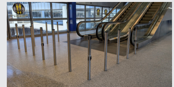
Our installers leave it better than they found it. No muss, No fuss.
